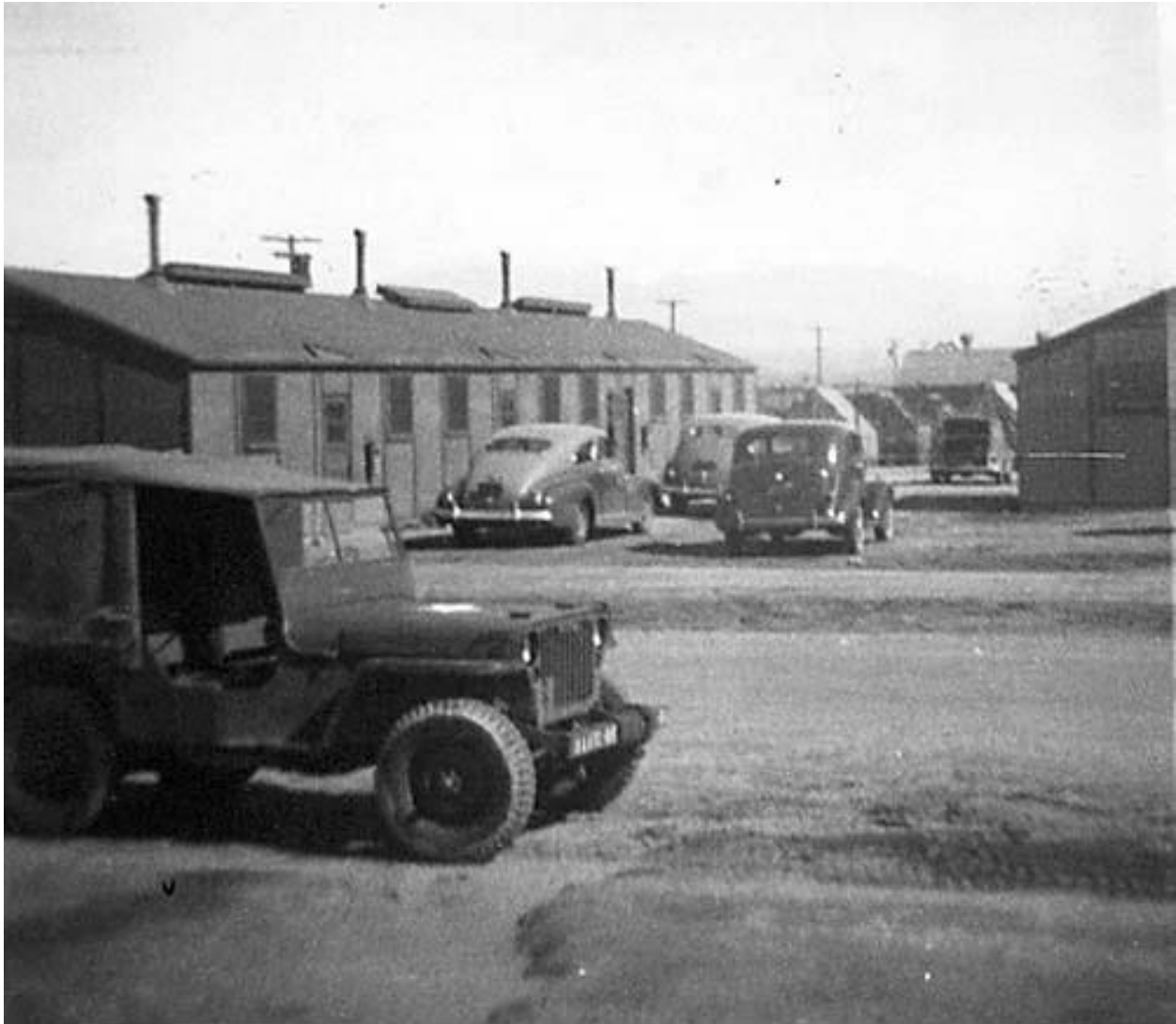
20. Mess Hall Building with Jeep in front.
