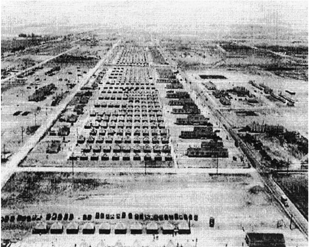
18. Aerial view of Camp Haan. Six-man huts in center, left of huts are latrines, and to right are mess halls and supply / day room buildings (SWP)
