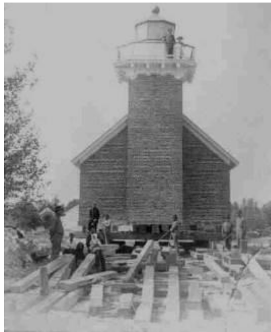
1890's picture of the Sand Point Lighthouse in Baraga being moved closer to the shore because it was built to far inland.
