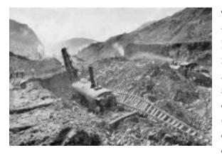
The French tried, and failed, to build a canal through Panama in the late 19<sup>th</sup> Century. The French design was a "sea-level" canal, which meant, essentially, a straight shot between the Atlantic and Pacific Oceans. This has some surface logic, since we might presume that neither ocean is on a higher elevation than the other. (Obviously, if one ocean were higher than the other, then the creation of a sea-level canal might create giant white-water rapids.)
