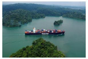
The Americans abandoned the sea-level canal and instead built a lake and a series of locks. The lake, Gatun Lake, is 85 feet above sea level. Ships entering the canal from, say, the Atlantic side, go through a series of locks and are ultimately raised to the level of the lake. After traversing the lake, the ships go through another series of locks and are ultimately lowered to the level of the Pacific Ocean.
